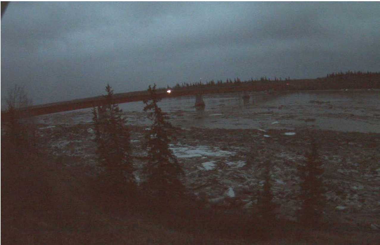
Only trace ice was observed passing by the Hwy 88 bridge near Fort Vermilion by 22:00 MST on April 30. The ice jam passed unimpeded downstream.
